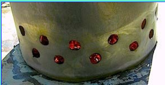
Air Intakes in Chimney smaller holes, wider distribution
